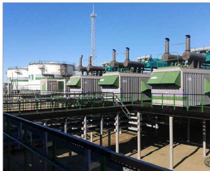
Cummins KTA50 gensets Cummins QSK60 gensets Prime power operation Natural Gas Extreme conditions – Siberia
